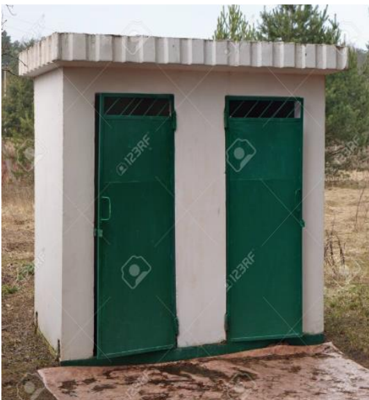
Pit Latrine Covered (without ventilation but covered/sheltered)
