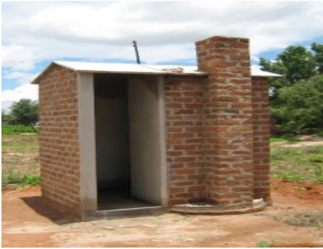
Ventilated Improved Pit (VIP) latrine 1
