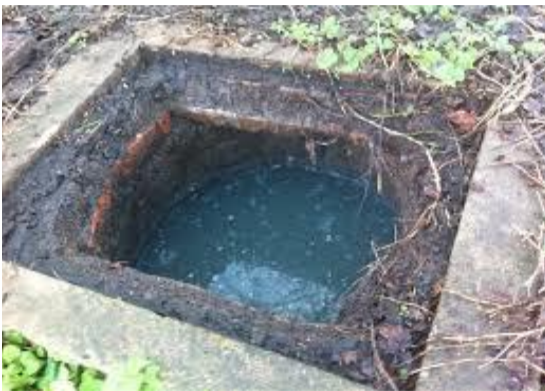
Cess Pool/ Cess Pit 2
