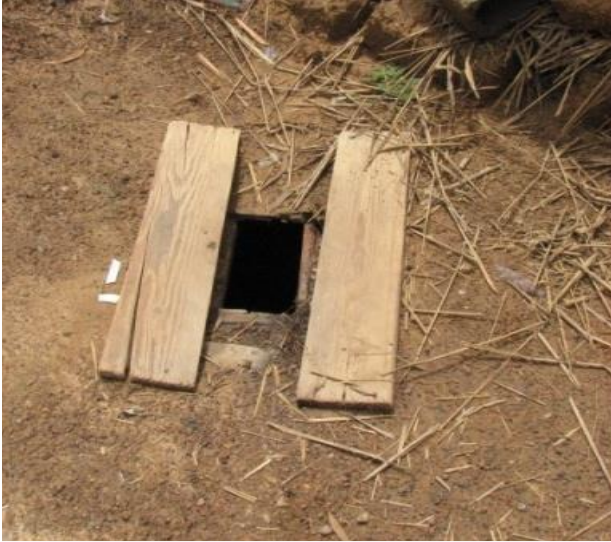
Holes/dug pits with temporary coverings or without shelter
