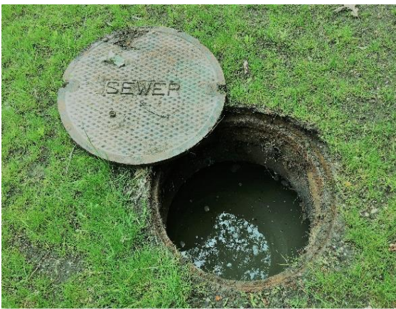
Cess Pool/ Cess Pit
