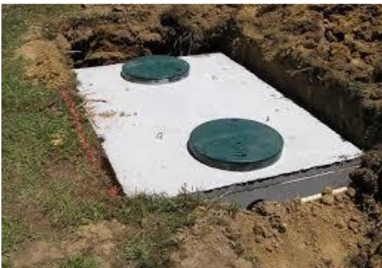
Concrete Septic Tank
